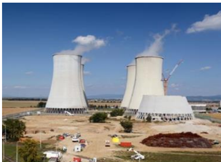
Figure 3 - Demolition of cooling towers.
